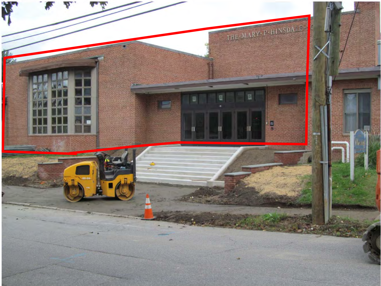
HINSDALE SCHOOL PORTIONS TO BE DEMOLISHED
