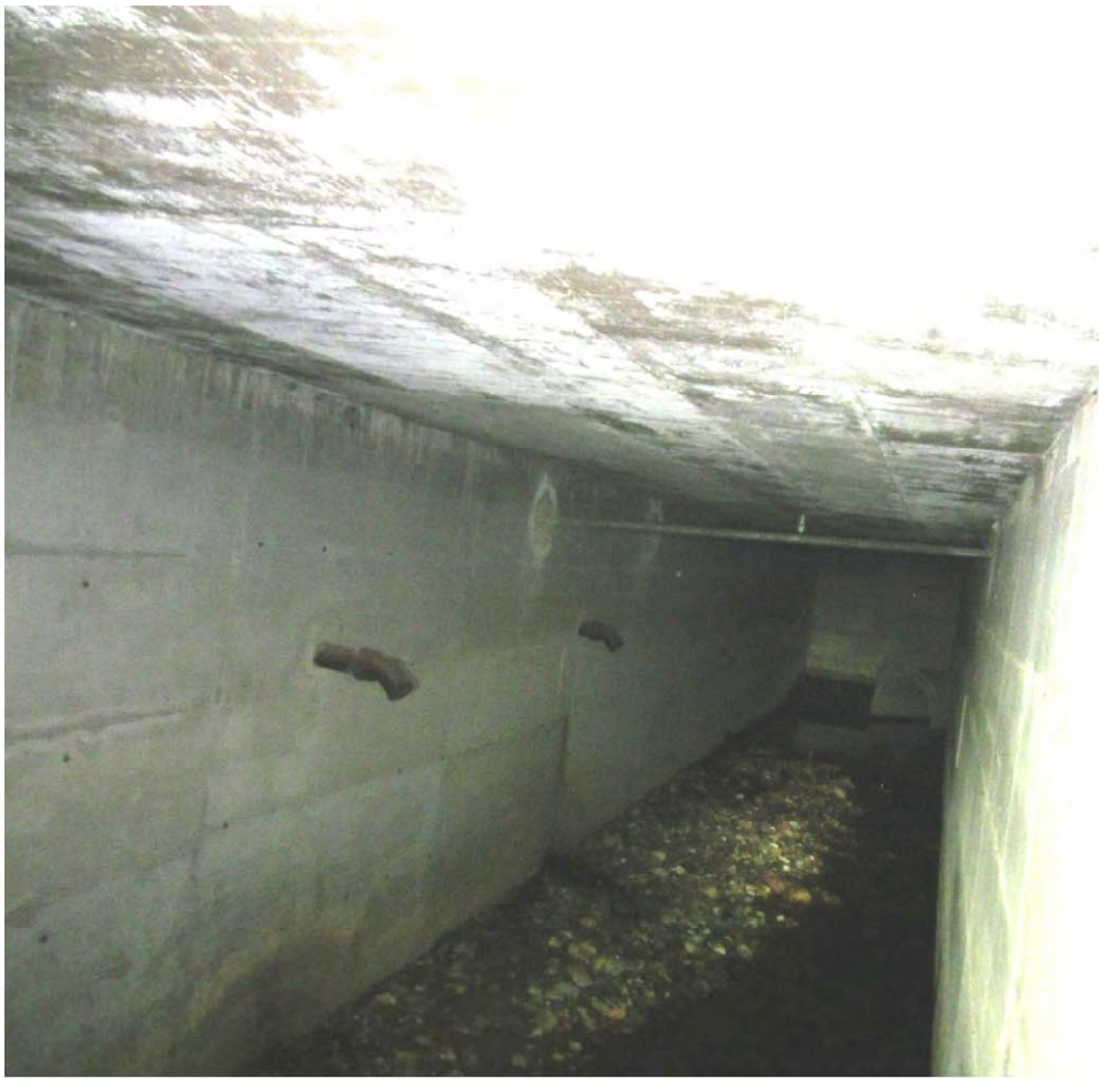
Culvert looking upstream
