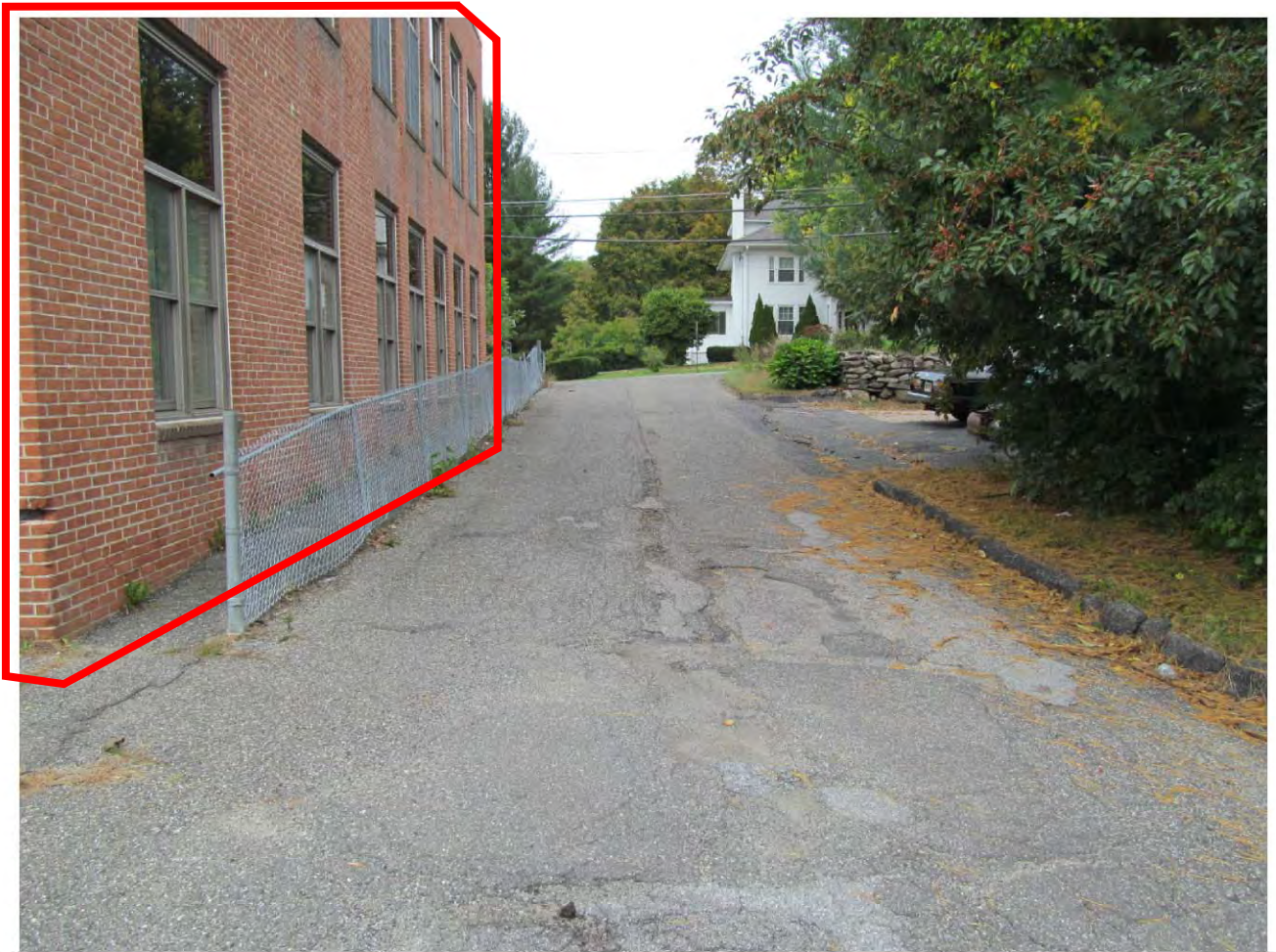
HINSDALE SCHOOL PORTIONS TO BE DEMOLISHED
