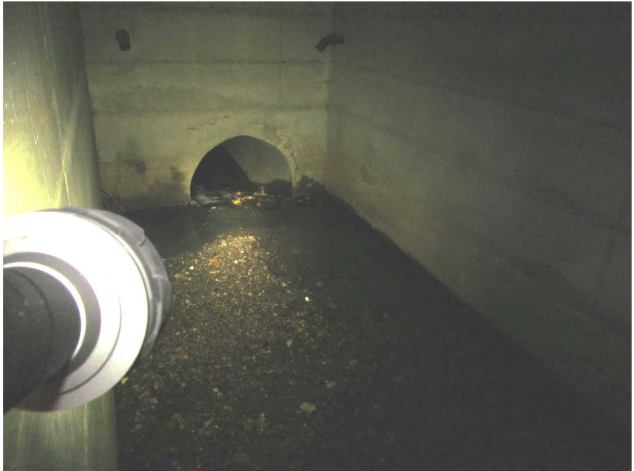
Culvert looking downstream
