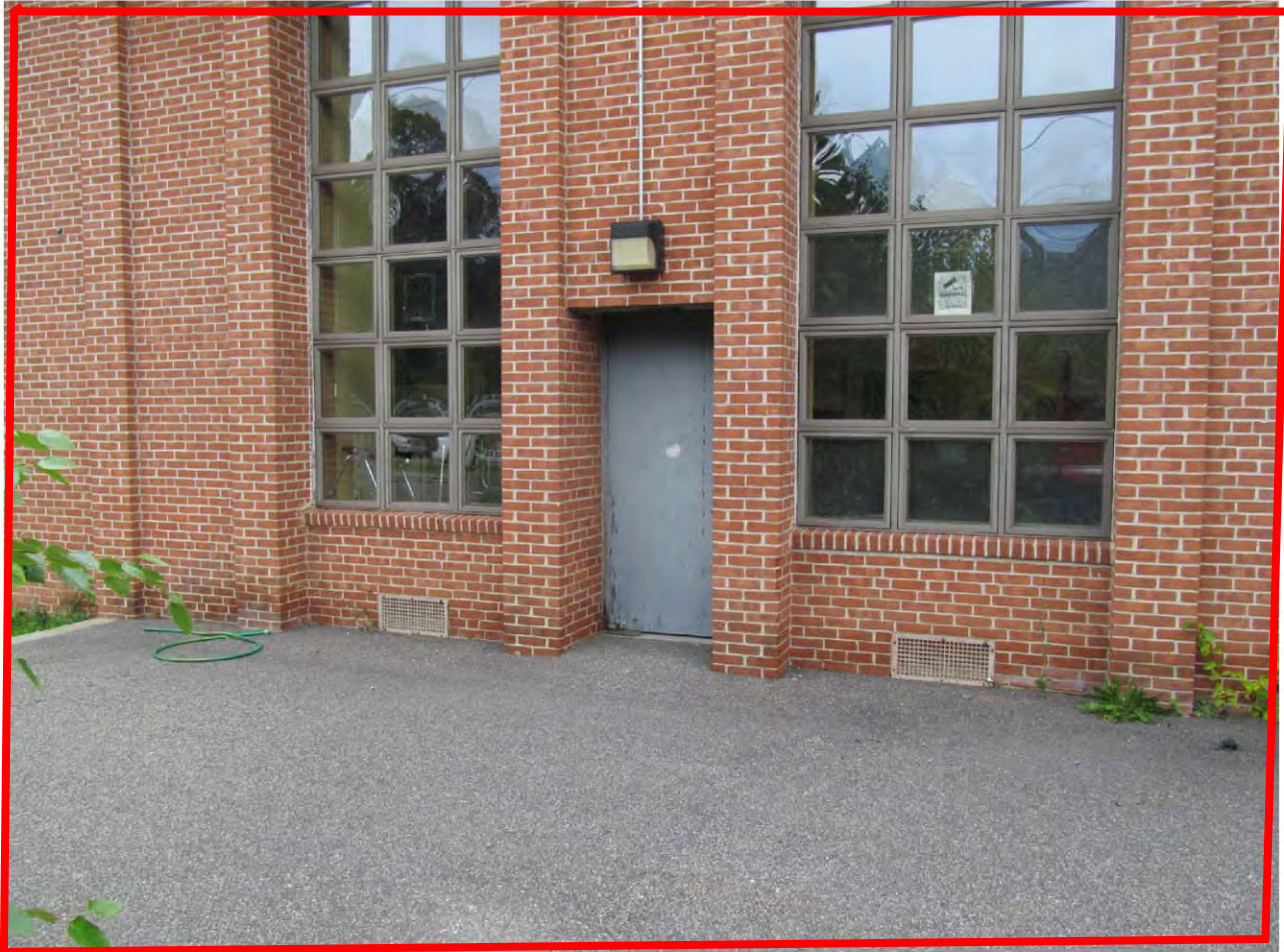
HINSDALE SCHOOL PORTIONS TO BE DEMOLISHED
