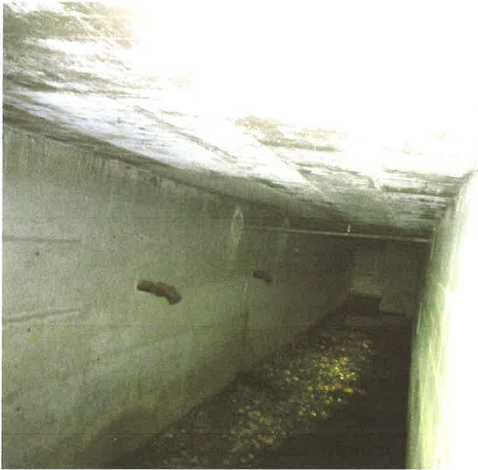
Culvert looking upstream
