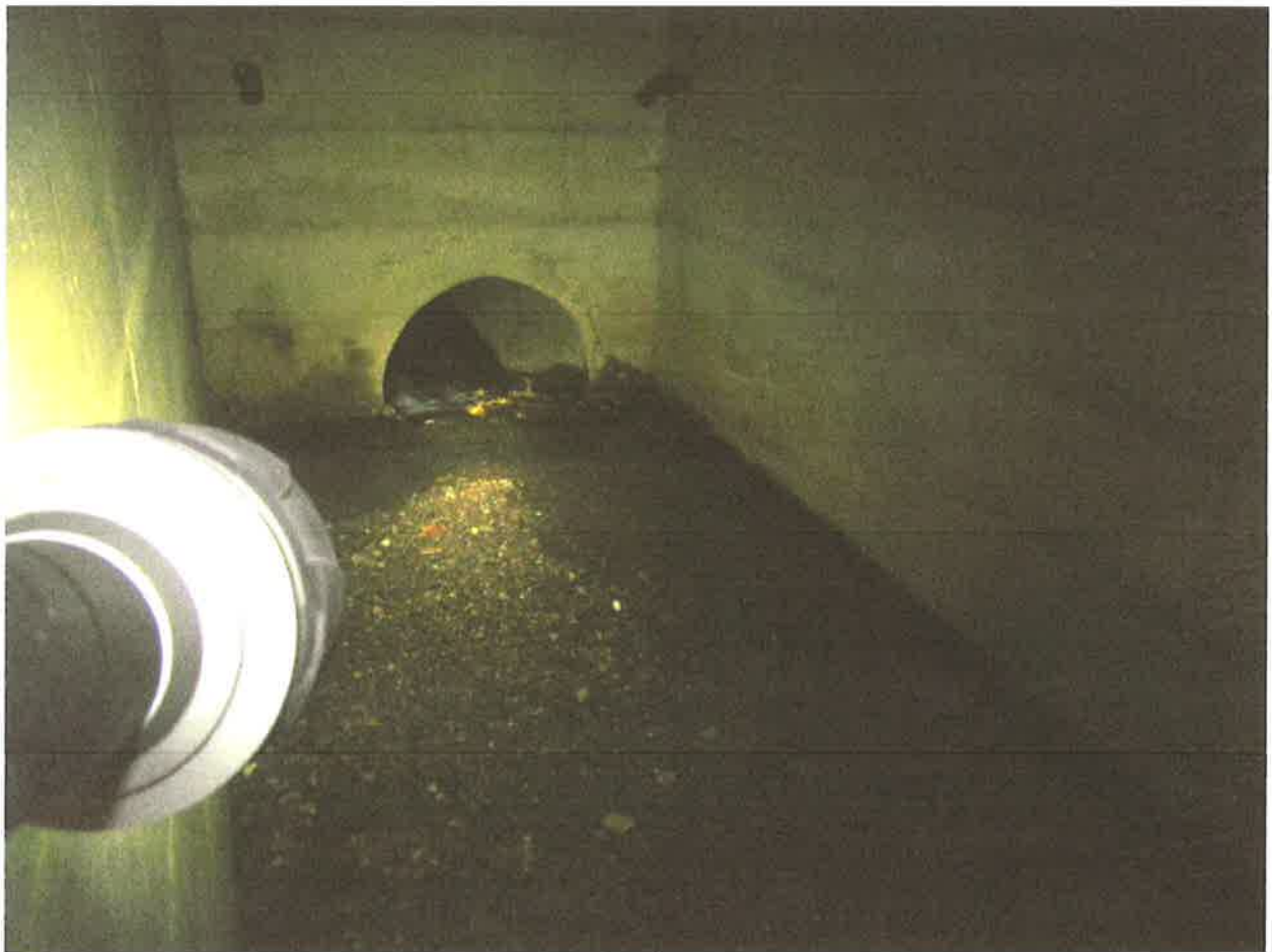
Culvert looking downstream
